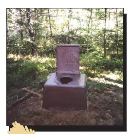
Figure 84—A fiberglass riser for a pit toilet in the Boundary Waters Canoe Area.
